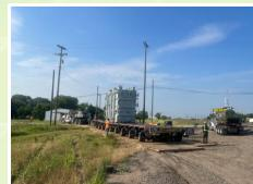
HLI railed this 351,320 lbs. transformer from Tula, Mexico, to a rail siding in Ponder, TX, where it was met by HLI's rigging crew. Upon arrival, the transformer was inspected for damage, before cutting the securements that had held it on its rail journey. The laying out of the jack-and-slide equipment commenced. The crew jacked the transformer up off the railcar, and transloaded the unit over to a waiting Goldhofer transport trailer.
