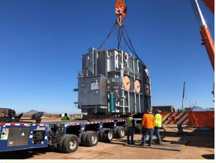
This job required the delivery of one 294,300 Lb. transformer from Laredo, TX to Buckeye, AZ. HLI was able to obtain all of the necessary permits and permissions to move the transformer from the transload facility, up to the final point of delivery inside the substation. Delivery was made easier by the use of an overhead crane, to lift the transformer from the railcar to the awaiting 19-axle girder transport trailer.
