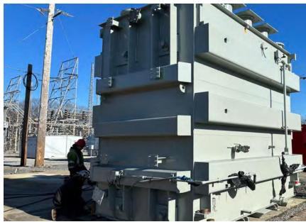
This job required the delivery of one 211,410 Lb. transformer from Laredo, TX to Port Jefferson, NY. First it was railed to Port Newark, NJ, where it was offloaded from the railcar, and then transloaded to a barge, to be barged to Port Jefferson, NY. Transloading the unit in Port Jefferson to the dual lane transport trailer was made easier using an overhead barge crane. With the transformer secured and safety checks approved, the journey to the customers substation began.
