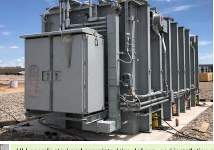
HLI coordinated and completed the delivery and installation of this 309,100 Lb. transformer from the manufacturer in Montgomery, AL to customers site in Mesa, AZ. After HLI's crew arrived at the rail siding, they began releasing the transformer from the railcar, to facilitate transloading to a dual-lane 19 axle girder trailer, for final delivery to the customers substation. The most efficient, and economical method for offloading the heavy transformer was by using the jack-and-slide system.
