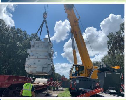
This job required the delivery of one 148,000 Lb transformer from Laredo, TX to Fort White, FL. HLI was able to obtain all of the necessary permits and permissions to move the transformer from the transload facility, up to the final point of delivery inside the substation. Delivery was made easier by the use of an overhead crane, to lift the transformer from the railcar to the awaiting 13-axle Perimeter Frame Lowboy transport trailer.
