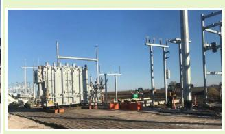
The crew jacked the transformer up off of the railcar, and used the slides to move the unit over to the platform trailer. Once loaded to the transport trailer, the transformer had a long haul to the final destination inside the substation. After a safe arrival at the substation location, it was removed from the transporter using the jack and slide system again. This put the transformer onto the final pad and after being rotated 90 degrees, it was ready for assembly and installation.
