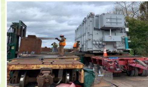
HLI railed this 414,000 lb. unit 1,057 miles from Montgomery, AL to a rail siding in Hopewell, NJ. After arriving at the rail siding, the transformer had to be offloaded from its heavy-duty railcar, to an over-the-road transport system, to be delivered to the customers substation. The best choice for offloading this heavy transformer from the railcar, and loading it onto the transporter, was using the jack and slide system.
