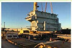
HLI was commissioned to move this 179,000 lbs. unit from customers site and deliver to a rail siding in Victoria, TX. After arriving at the customers site, the transformer was freed from its storage location, while two cranes were assembled to lift the transformer to a road transporter. Once successfully lifted, it was secured to the road transporter and began its journey to the awaiting railcar at the rail siding.
