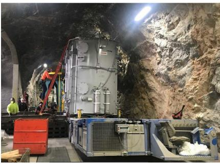
This project was especially technical, as it involved the partial dismantling of the old transformer and its removal from a tunnel, before transporting it to a temporary storage area for later pickup. The next phase was to stage the rigging gear at the pickup location for the replacement transformer, to enable it being transferred to a specialized Goldhofer transporter for its final transportation to the tunnel entrance, along with its auxiliary parts.
