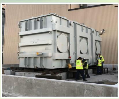
Upon safe arrival at the substation, HLI's crew offloaded the unit from the Goldhofer trailer onto the final installation pad, using the jack and slide system. HLI's crew then unloaded three loads of accessories and finally conducted a megger testing of the unit, all results were within the necessary parameters set by the manufacture.
