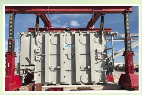
After inspection of the transformer, it was lifted off the rail car, and placed on the transporter to haul to its destination. After a safe arrival at the substation location, it was removed from the transporter using the Gantry equipment. Once the transformer travelled over the pads retaining wall, it was set on slide rails and slid over to its final installation pad.
