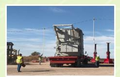
HLI railed this 257,530 lb. unit from Eagle Pass, TX to a rail siding in Dodge City, KS. After arriving at the rail siding, the transformer had to be offloaded from its heavy-duty railcar to an over the road transport system to be delivered to the substation. HLI chose to use Gantry equipment for offloading this heavy transformer. The Gantry equipment had to be assembled and disassembled a number of times during the various stages of this move.
