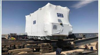
The crew jacked the transformer up off the railcar and used the slides to move the unit over to the special trailer. Once loaded to the transport trailer, the transformer was transported to its destination inside the substation. After a safe arrival at the substation location, it was removed from the transporter using the jack and slide system again. This put the transformer onto the final pad ready for assembly and installation. The job was completed on time and on budget.
