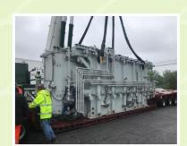
Two 231,000 Lbs. transformers crossed the border from Mexico to the United States via HLI's Laredo, TX transload facility. From there HLI railed them to a rail siding close to their future home in Carlstadt, NJ. The rigging crew met the units at the rail siding with an all terrain crane and loaded it to a transport trailer.
