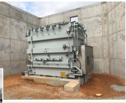
HLI railed this 168,484 lbs. transformer from the nearest rail siding in Lynchburg, VA. Once arrived at the rail siding, the transformer had to be offloaded from its heavy-duty rail car to an over the road transport system to be delivered to the substation in Lynchburg. The best choice for offloading this heavy transformer from the rail car and loading the large transporter was using a jack and slide system.
