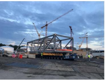
HLI was requested to relocate 10 prefabricated pipe racks, weighing up to 225 metric tons each, at a site in Jessup, Pennsylvania. The pipe racks were 8.22 m wide x 9.75 m high and 28.9 m long. HLI provided all the jacking, transportation equipment, qualified personnel and obtained all permits.
