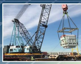
HLI picked-up three transformers from the Port of Newark, NJ. The transformers arrived at the Port of Newark in a heavy lift ship where the securing were cut loose from the units. A 1,000 ton barge crane, was contracted to lift the transformers from the ships hold and transfer them to an awaiting railcar. Once they were placed on the railcar, HLI's crew started to fabricate hold down brackets to facilitate a safe journey.
