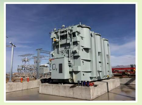
The transformers were moved to the girder trailer, using a jack and slide. State police then provided an escort to the substation. Once inside, the substation, the transformers were slid out of the girder trailer to a crib pile, they would then be rotated and slid on to their final pads. Units were tested, and found to be within set parameters. Accessories were then unloaded. The entire job was completed safely and on time.
