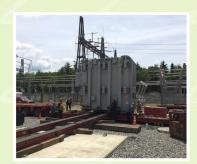
HLI utilized ocean freight from Brazil to the Port of Baltimore, it was then transferred to rail, arriving at a rail siding in Otter River, MA. After arriving at the rail siding, the transformer was offloaded from its heavy duty rail car to an over the road transport system to be delivered to the substation. Jack and slide was utilized to transfer the transformer from the railcar to trailer.
