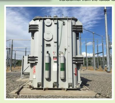
The crew jacked the transformer up off of the car, and used the slides to move the unit over to the platform trailer. Once loaded to the transport trailer, the transformer was transported to its final destination inside the substation. After a safe arrival at the substation location, it was removed from the transporter using the jack and slide system again. This put the transformer onto the final pad. Once installed, the unit was tested successfully.
