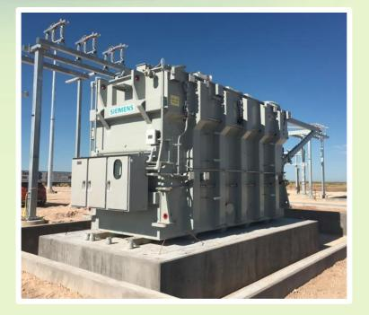
They positioned hydraulic slide beams beneath the unit and safely loaded it onto a specialized transport trailer, before hauling it to the final site. HLI's crew mobilized to the site and offloaded the unit from the transport trailer, using the jack and slide method. The unit was then spun into its proper orientation on its pad, and then bolted down.
