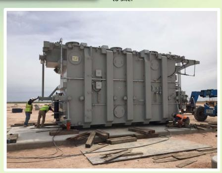
The crew accomplished the haul to site without incident and positioned the trailer near the final pad for offloading. They jacked up the unit to pad elevation and slid it across onto the receiving concrete surface. They used a turntable to rotate the unit to the proper orientation and jacked it down to rest on the final pad. The accessories were offloaded nearby to await final installation.
