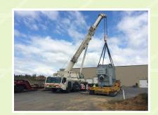
This 172,100 lbs transformer crossed the border from Mexico to the United States at HLI's Laredo, TX transload facility. From there HLI railed it to a rail siding close to its future home in Decatur, AL. The rigging crew met the unit at the rail siding with an all terrain crane and loaded it to a transport trailer.
