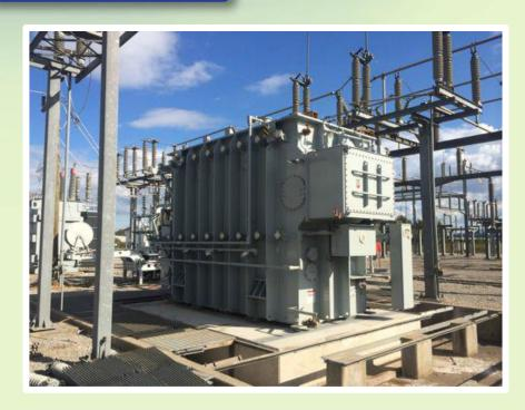
Once it had been transloaded, the transformer traveled a short distance over roads to the substation it had been manufactured to join. At the final site, the crew used the same all terrain crane to lift the unit off the transport trailer and set it safely on the customer's pad. With the delivery completed, the transformer awaited final assembly.
