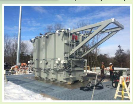
Once the roads had been cleared the next day, HLI commenced the road transport and hauled the transformer 12 miles to the site. At the substation, HLI used a jack and slide system to move the unit from the transport trailer onto the customer's final pad. The entire project was completed safely and on time.
