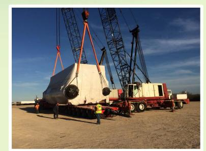
With everything prepared for the second lift, HLI maneuvered the receiving Goldhofer to a position adjacent to the boiler. The two cranes lifted in unison from either end of the unit until it had reached a sufficient height to allow the Goldhofer to sneak in beneath it. The crane carefully lowered the boiler onto the deck of the transport trailer where it would be secured and hauled to its final location.
