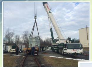
The crew carefully hauled the transformer the short distance from the rail siding to a nearby storage yard where the unit would reside until it is needed. Once adjacent to the temporary receiving pad, the crane lifted the transformer again, this time off the trailer, and placed it gently onto the pad. The entire job was completed safely, within schedule, and without incident.
